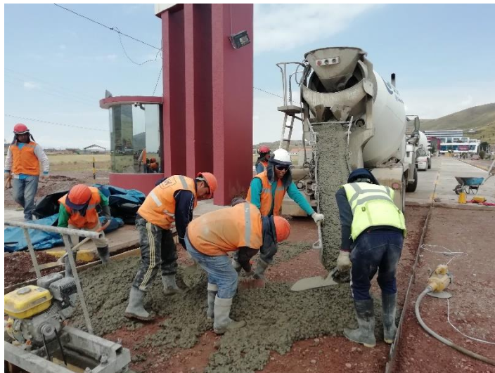
Figura 26. Colocado del concreto MR=48\text{kg/cm}^2 – F^{\prime}c=350\text{kg/cm}^2
