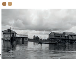
1 Calle las Flores Sector N° 11, partially flooded, at 40 cm of ground surface. During 15 days in March, the flood covered a distance of 60 m from the initial point shown.
