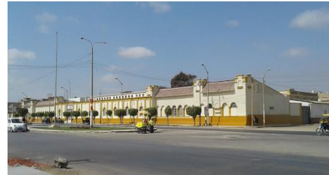
Figura 86. Hospital Belén de Lambayeque
