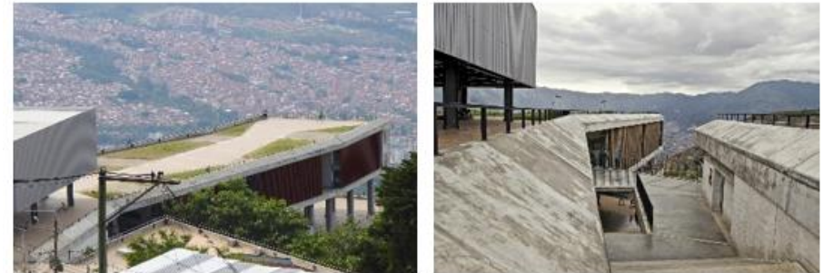
Figura 72: Vistas del colegio Antonio Derka. ArchDaily.
